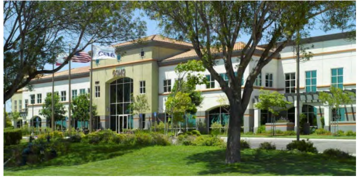
Pictured: GSMS, Incorporated facility in Camarillo, California
