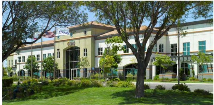
Pictured: GSMS, Incorporated facility in Camarillo, California
