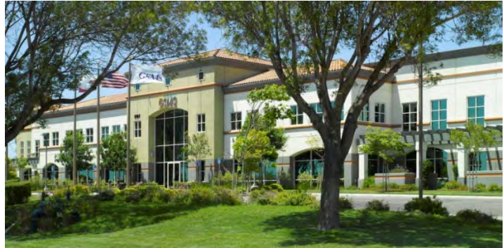
Pictured: GSMS, Incorporated facility in Camarillo, California
