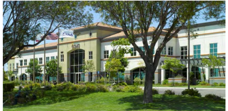
Pictured: GSMS, Incorporated facility in Camarillo, California
